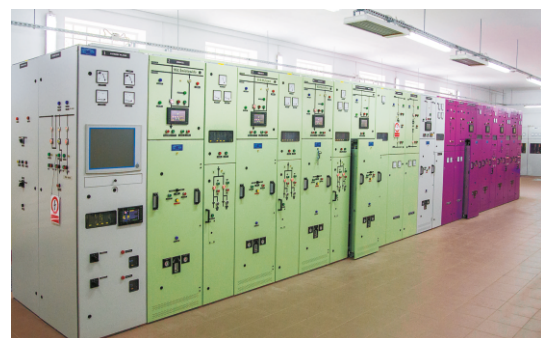
Train 3 kV DC switchgear for traction power substation
