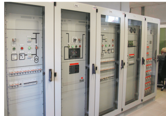
CZAT7 automation in the gamma filter field
