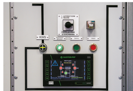
CZAT7 controller, with the CZAT Synoptic HMI panel, in the auxiliary switchboard 400 / 230V, realizing the control remote and automatic transfer switching (ATS)
