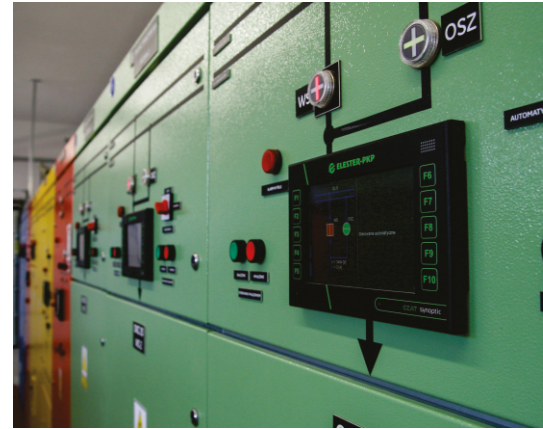
CZAT7 and HMI device CZAT Synoptic in the traction or backup feeder field - DC power substation Łachów
