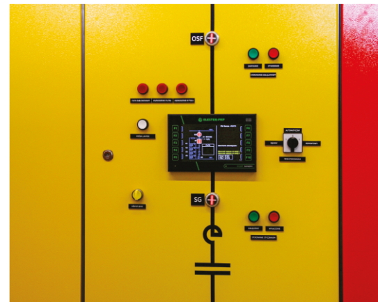
CZAT7 automation in the gamma filter field
