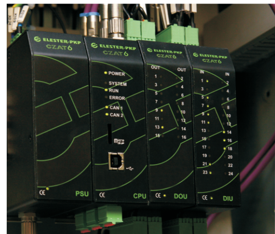
CZAT 6 in the traction feeder field
